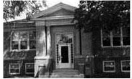
Janesville Free Public Library, 102 W. 2nd Street, Janesville, MN, built in 1912, Architecture: Classical Revival
