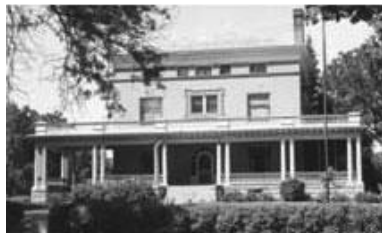
John W. Aughenbaugh residence, also known as the Masonic Temple, 831 NE 3rd Avenue, Waseca, MN, built in 1897 Architecture: Renaissance-Revival
