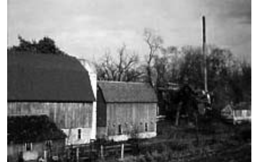
Seha Sorghum Mill, County Highway 5, Janesville, MN, built in 1890s
