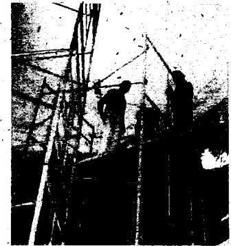
Don Wynnemer and George Kastelle putting up the scaffolding.
