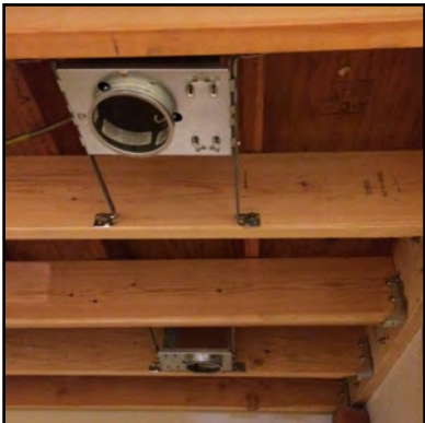
Light fixtures in place!
